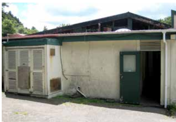
Example of unlit rear of a bar
